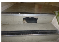
Damaged floor tile on stairwell
